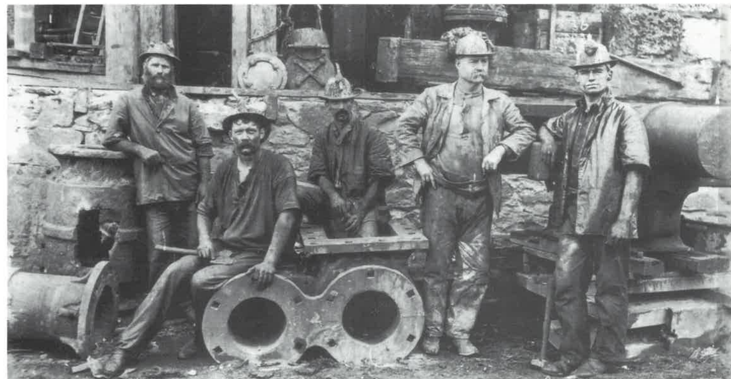
Miners clothes were made of heavy drill; resin hardened felt hats protected their heads and a candle provided light underground. The candle was attached to the brim of the hat with a lump of clay - spare tallow candles hung by the wick around his neck.
